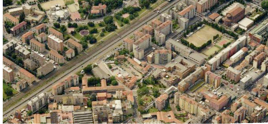
The subway line combined with a fast traffic road create a strong physical barrier that divides the district
