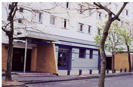
The renewal of this social housing created premises at the ground floor to provide information and assistance to the tenants © IAU île-de-France
