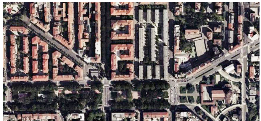
This public housing project built in the 50's is admirably well integrated in the surrounding urban pattern
